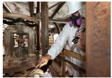
ASBESTOS CONTAINMENT AREAS
