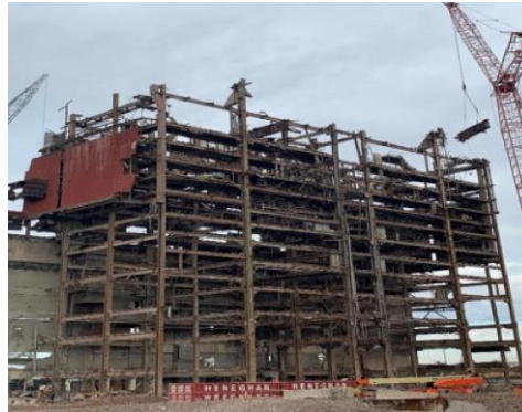
DECONSTRUCTION Mechanical • Dismantle • Recycle/Dispose
